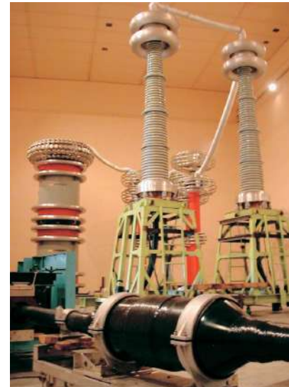
61kV withstand voltage testing
