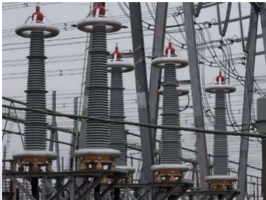
Scene after completion of outdoor terminal insulator assembly of UHV substation
