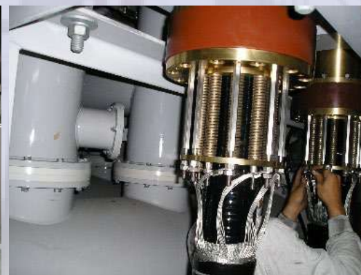
Hua Ho's engineering technicians were performing terminal assembly at the substation
