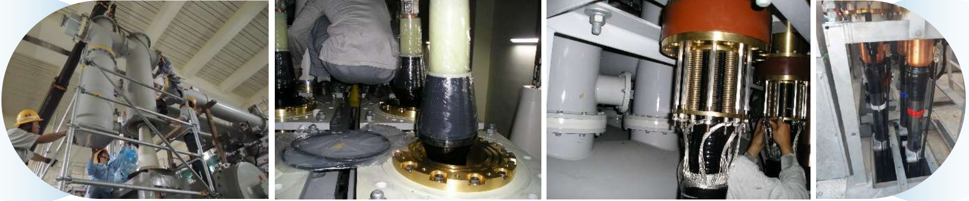
Hua Ho's engineering technicians were performing terminal assembly at the substation
