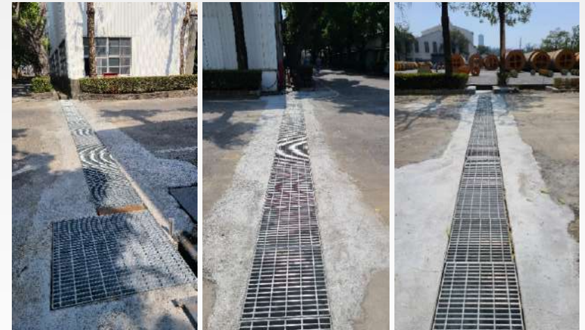
Sequential clearing and maintenance of the plant's drainage channels.
