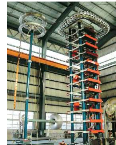
345kV ultra-high voltage cable partial discharge testing
