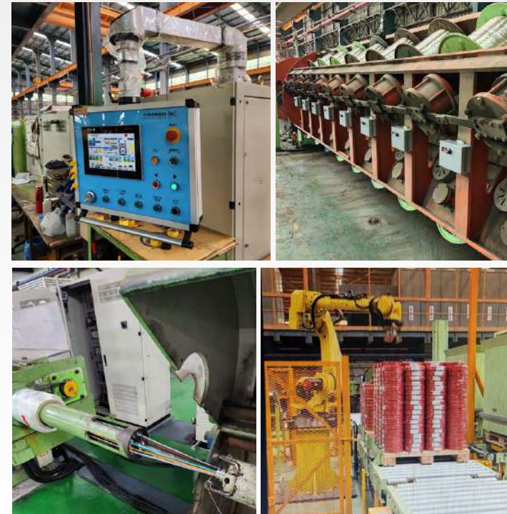
Increased risk of downtime for aging equipment.
