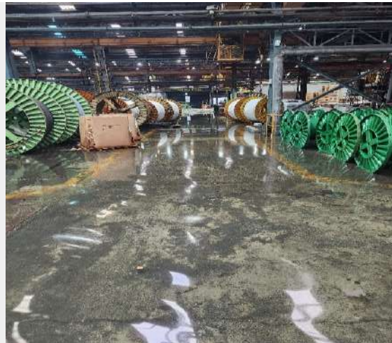
PCV25-2 medium-voltage CV cable coiling area
