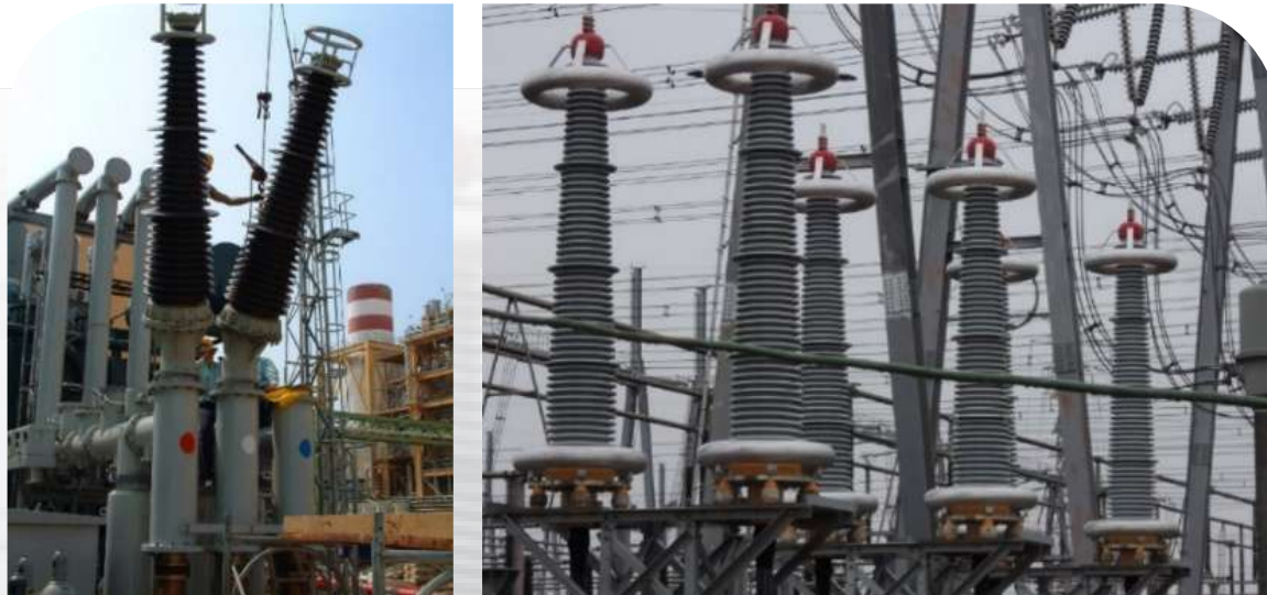
Outdoor construction of the UHV substation Scene after completion of outdoor terminal insulator assembly of UHV substation
