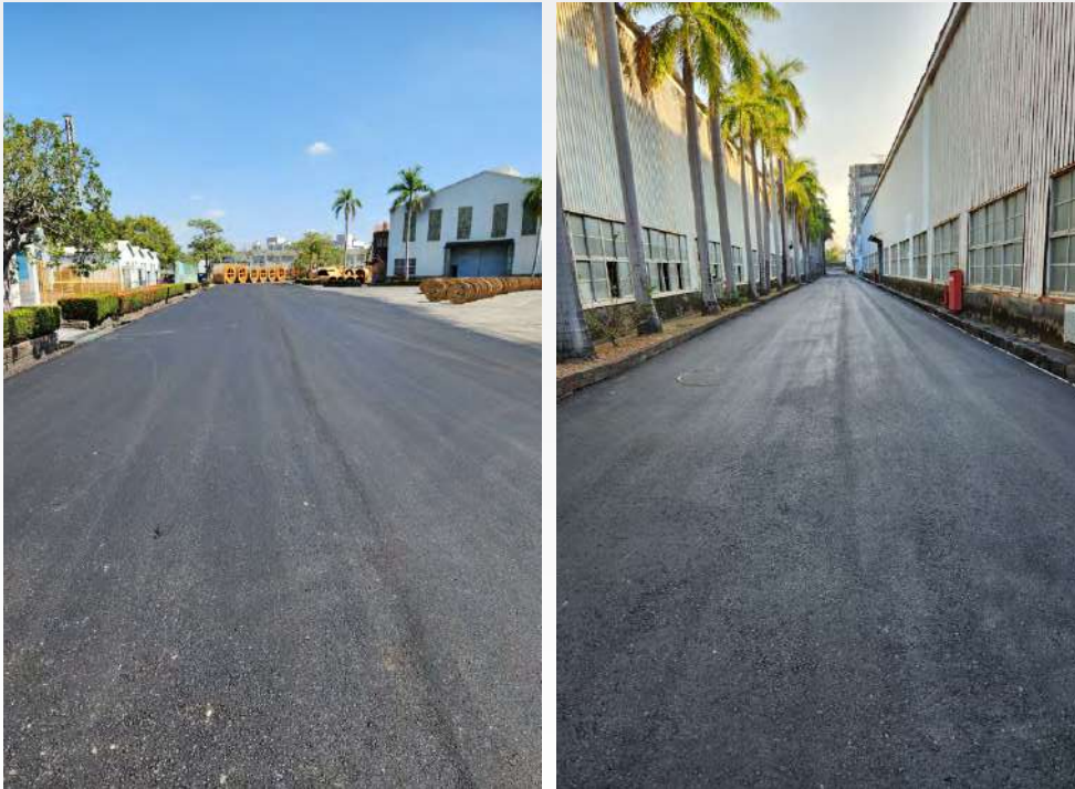
Pavement repair project at the Kao-Nan Plant and parking lot.
