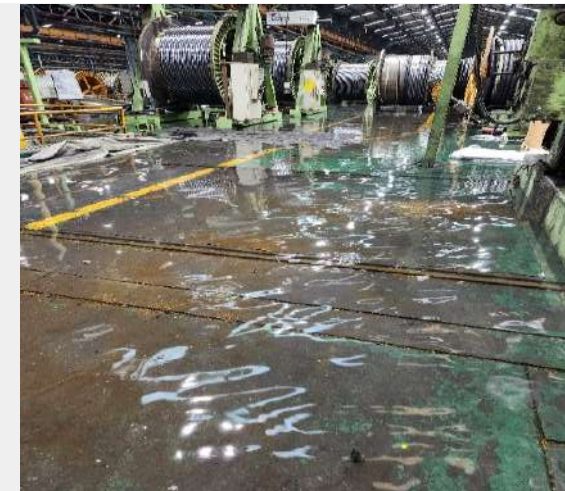
PCV25-2 medium-voltage CV cable coiling area
