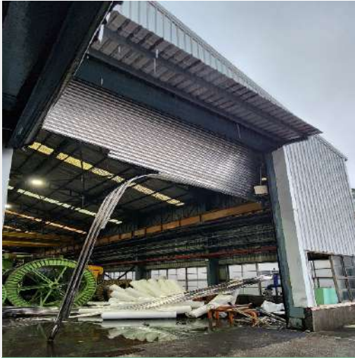
PE150 north-side rolling door
