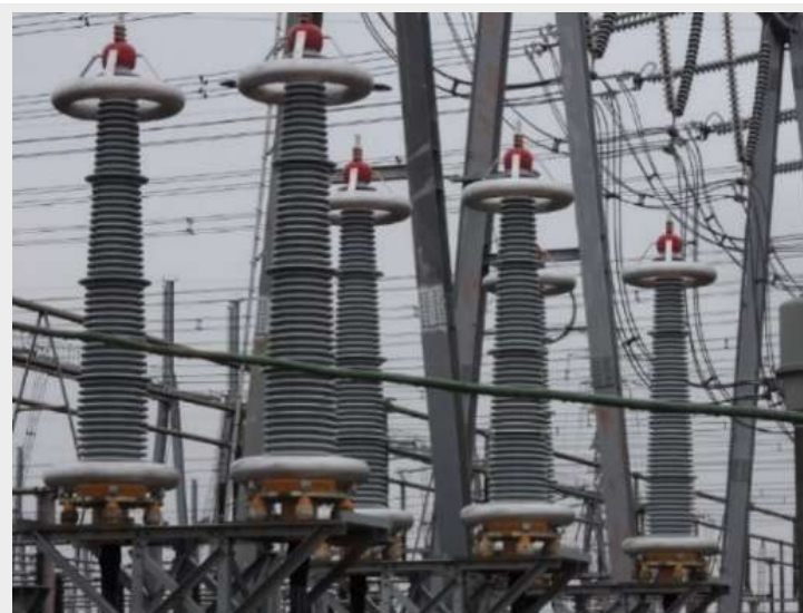
Scene after completion of outdoor terminal insulator assembly of UHV substation
